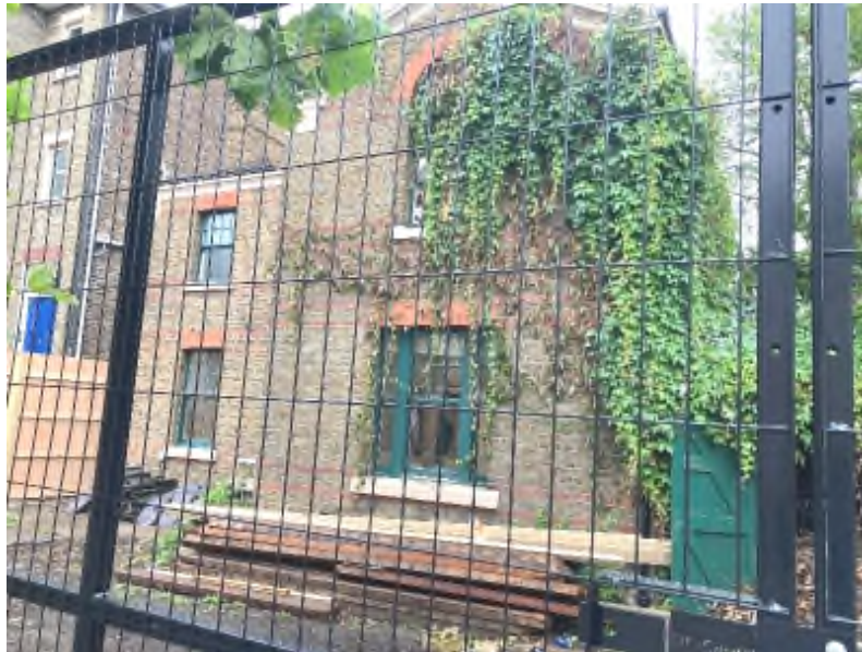
No. 156 Junction Road, during demolition in July.
